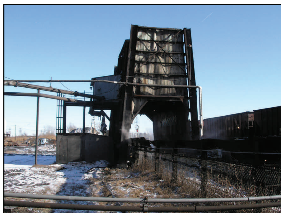
East Quench Tower that required the installation of baffles for particulate emission control per the Title V air permit
