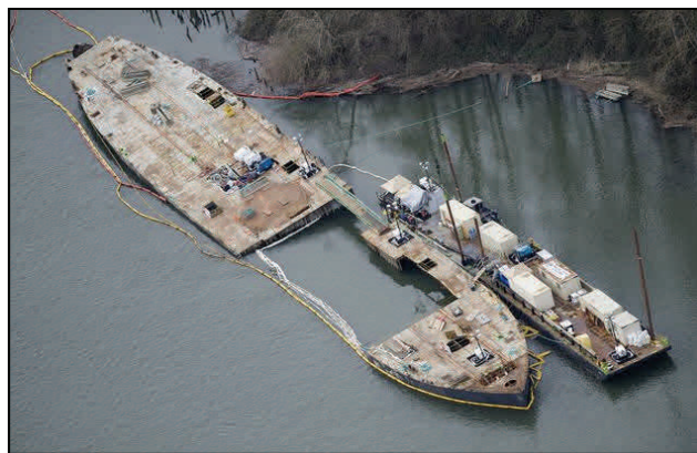
Aerial view of the M/V Davy Crockett surrounded by a cofferdam and dismantled in place.
