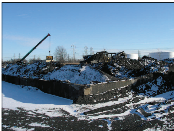
Coal tar concrete pad where decanter tank tar sludge (K087 - listed hazardous waste) should have been mixed with coal prior to placing the mixture into the coke oven battery
