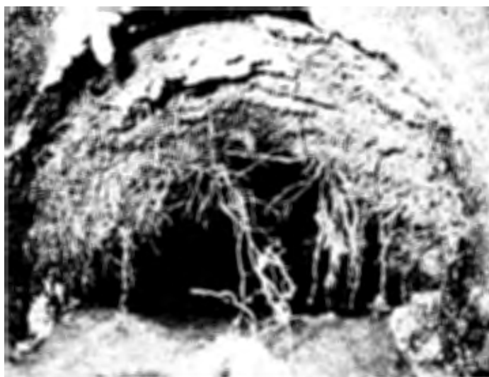
Figure 2. Roots in Murray Run Interceptor
