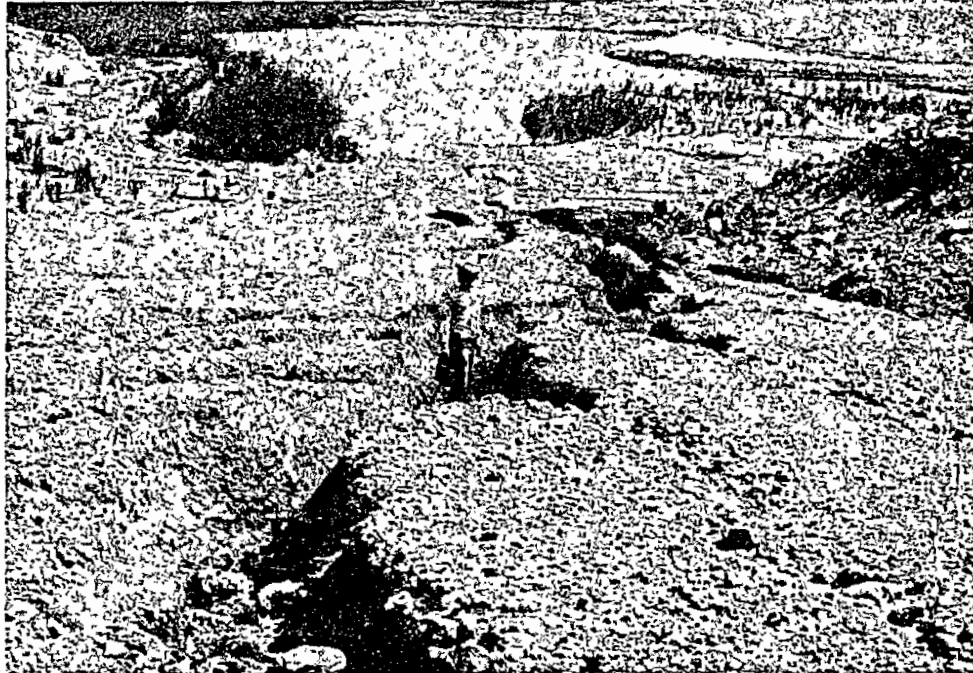
Figure 6.10 Recent erosion of unstabilized overburden piles at the inactive Galen mine, Karnes County, Texas
