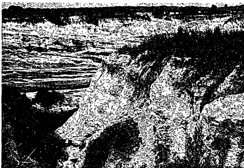
Figure 6 13 Overburden pile showing the weak vegetative cover and gulying associated with improper stabilization at the Manka Mine, Karnes County, Texas. Mine stabilized in 1974
