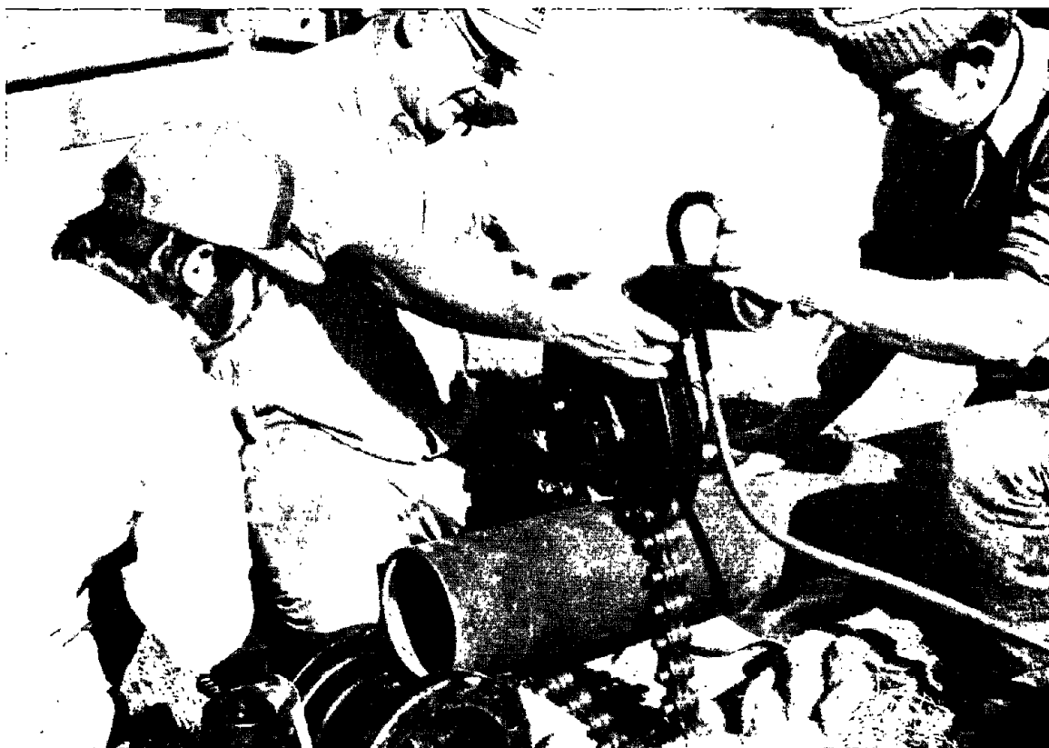
Figure 8. Problems were encountered in cutting pipe supplied under contract. The supplied pipe was not cast iron but a more durable and stronger, mild steel. The hydraulic pipe cutter operates only on brittle pipe.
