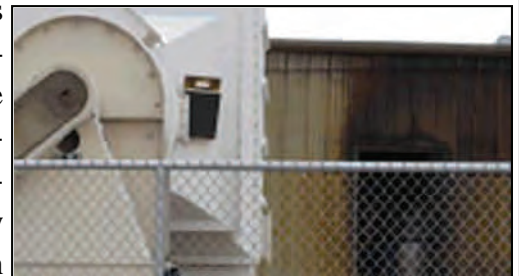
Building with heavily stained exterior as a result of the nitrogen oxide fumes.
