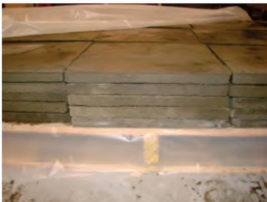
Figure 5. Concrete Curing
