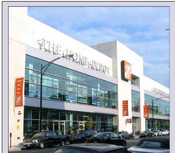
Exhibit 7. Home Depot in Chicago. Home Depot opened a two-story store that fronts North Halsted Street in the Lincoln Park neighborhood of Chicago. It not only changed the conventional layout of its store to fit the setting, but it also carries a different mix of merchandise designed to meet the needs of urban residents. Photo source: Payton Chung via flickr.com.
