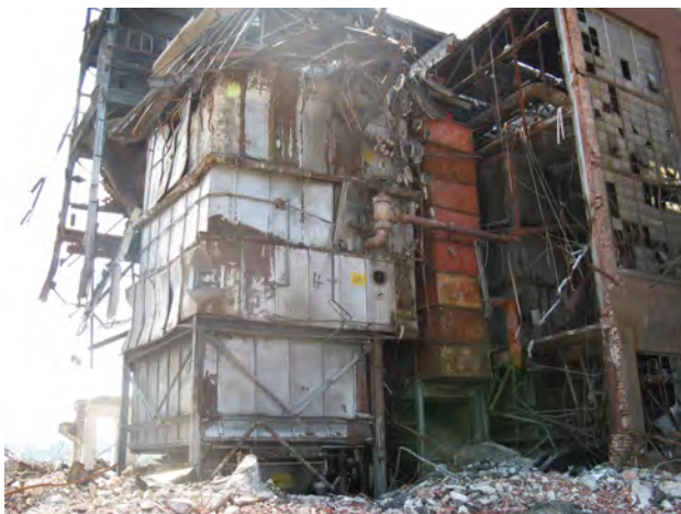
Stripped boiler from powerhouse of the facility
