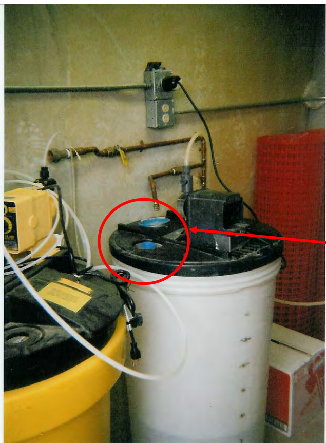
Exhibit 4.8 Example of an Air Gap on a Chemical Feed System
