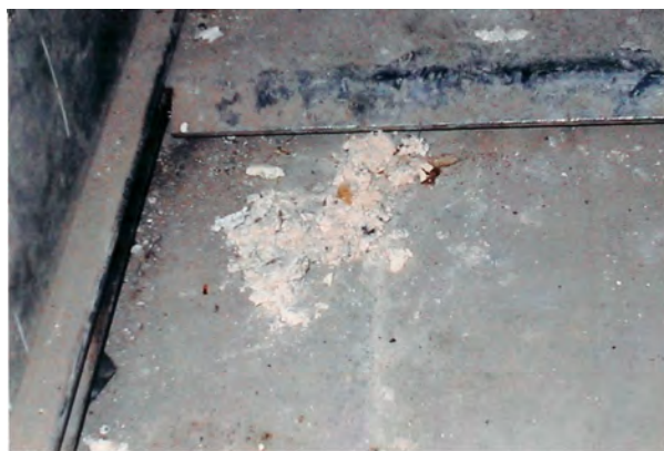
Regulated asbestos containing material pipe insulation debris.
