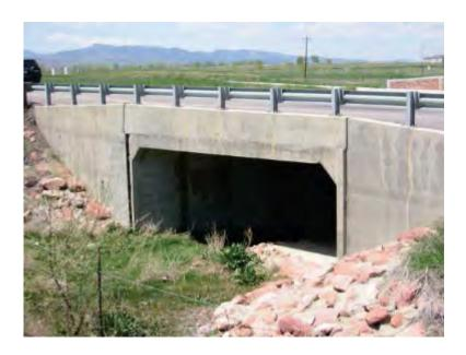
**Figure 3-2 Concrete Box Culvert**
