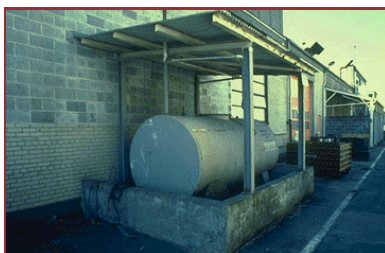
7 - Covered AST with secondary containment (above)
