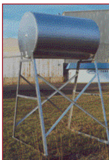
7 - Covered AST with secondary containment (above)
