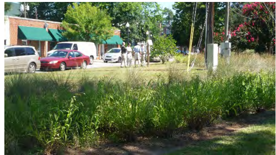
Exhibit 25. Rain gardens in street medians help manage stormwater while providing attractive landscaping.
