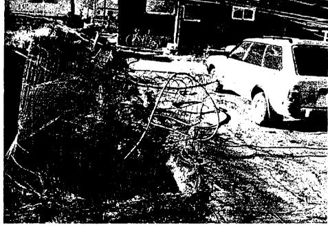
Hazardous Opening Caused By Shaft or Rise Failure
