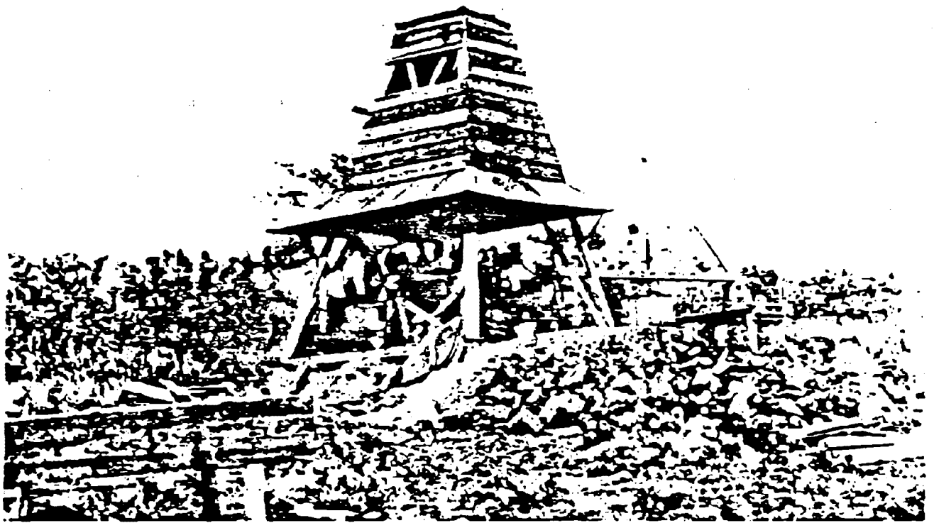
Between 1901 and 1907 more than twenty-five hundred shafts were sunk in the Wichita Mountains. Most were crowned with horse-powered hoists and shaft houses, such as this one near Snyder. Courtesy Western History Collections, University of Oklahoma Library.
