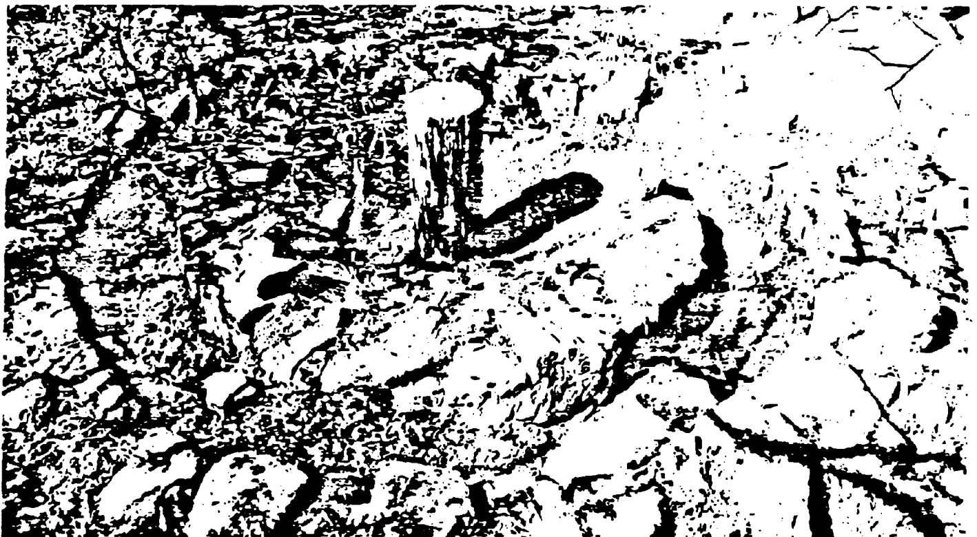
In 1901, William Larve, known as "Dutch Bill," who mined thirty years in the West and Mexico, built this Spanish-type arrastra just east of Mount Shendan on Cedar Creek. It is typical of many crude ore grinders found over the state. The rock was crushed by drag stones pulled round and round by burros.
