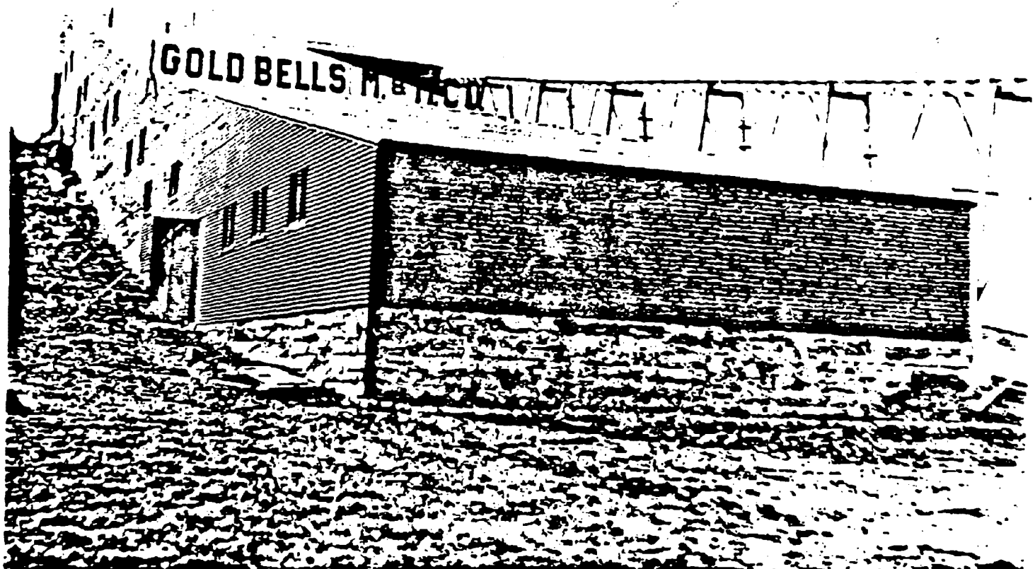
Begun in 1904, this fifty-ton cyanide processing plant one mile south of Wildman was erected by Wildman's founder, E. A. Williams, at a cost of seventeen thousand dollars. The tramway led from the ore mill to the Gold Bell Mine, a quarter of a mile away. Courtesy Hugh Corwin.
