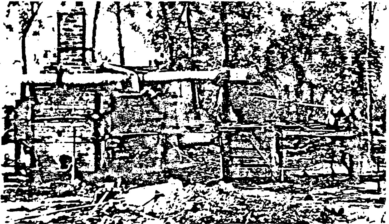
Virtually every mining camp in the Wichitas had its own furnace for smelting ore. In 1906, Olive Wells completed this four-ton, nine-foot-high test smelter at Golden Pass, north of Cache. Courtesy Bert Cook.
