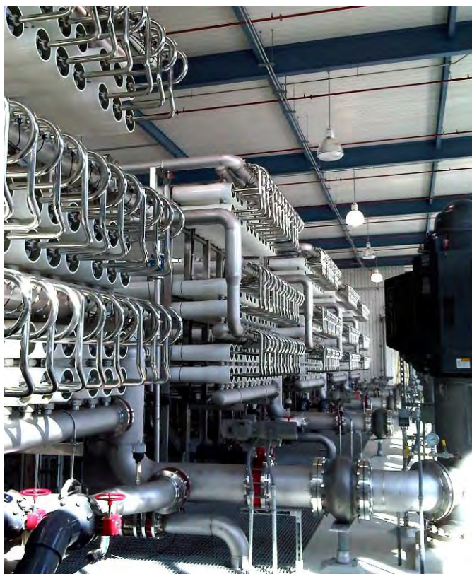
Figure F-2. Photograph of reverse osmosis system.
