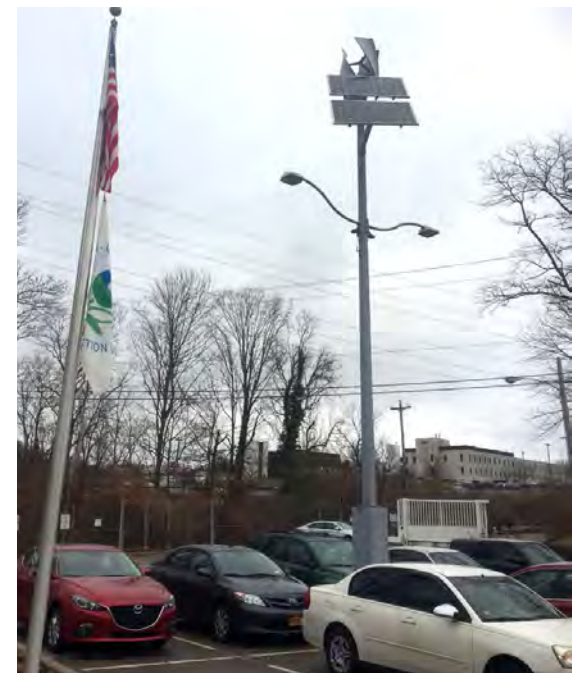
The Center Hill Facility installed a solar/wind-powered light as a prototype in its parking lot. The light has performed well. In its first year of operation, it generated 357 kWh, which exceeded the amount of energy (267 kWh) that it used to illuminate the parking lot.
