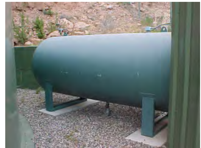
A Metal Storage Tank
