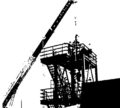
Figure 3-8. Vessel installation at CE-CERT's Hynol test facility.
