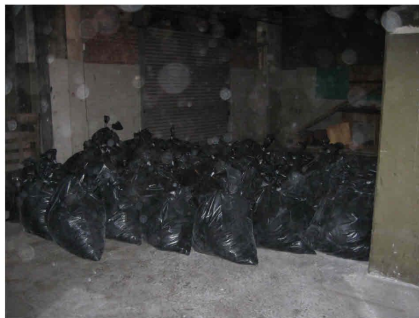
Inside warehouse —bags full of friable asbestos. The asbestos in the dumpster was bagged by workers, then moved into warehouse.
