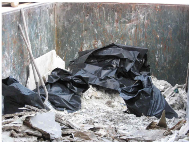
Dumpster containing friable asbestos. NYS-DOL inspector observed two unprotected workers inside this dumpster, including a 16 year old.
