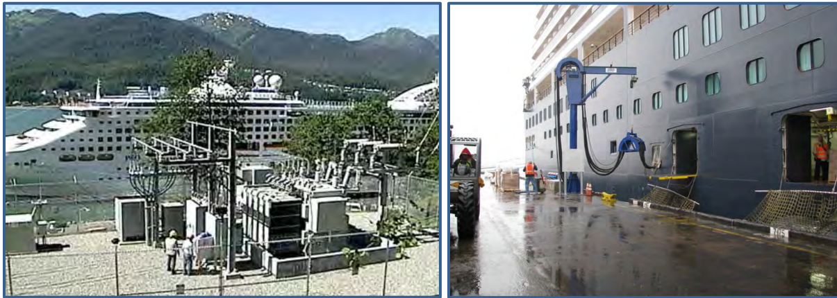
Figure 1: Electrical substation (left) and high voltage shore power vessel connection system (right) Source: Port of San Diego
