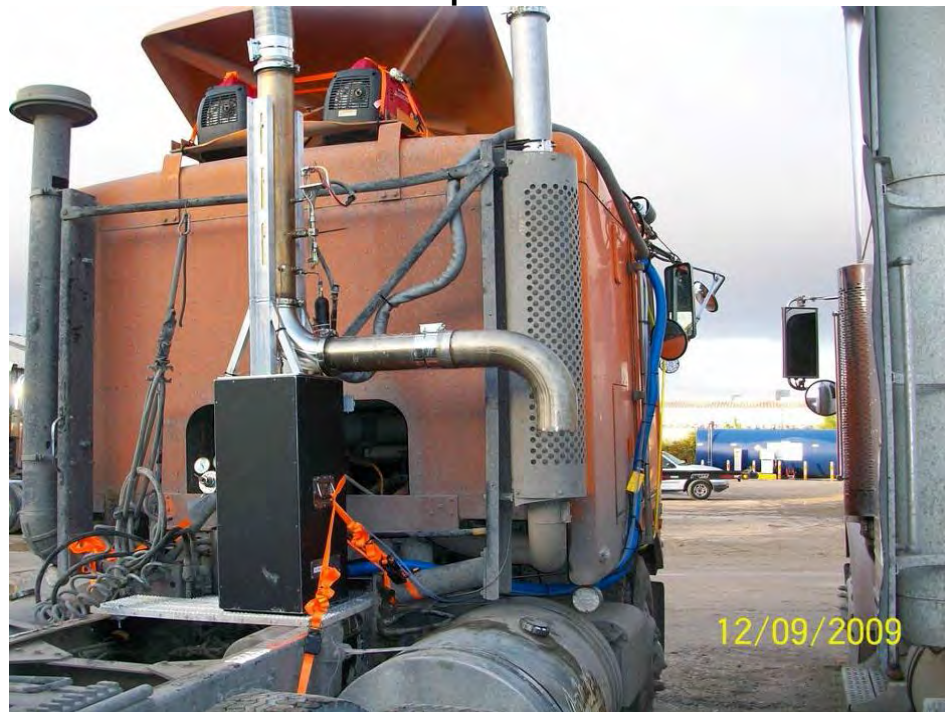
Figure 5.1-2 PM/Gaseous Test Components with Generators on Roof
