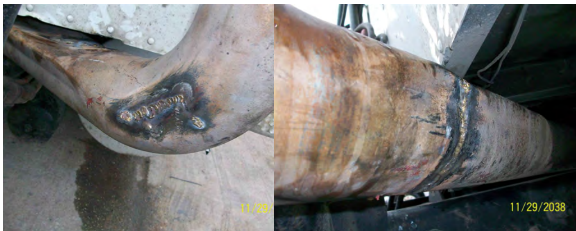
Figure 8.2-1 Exhaust System Repairs Performed During Study
