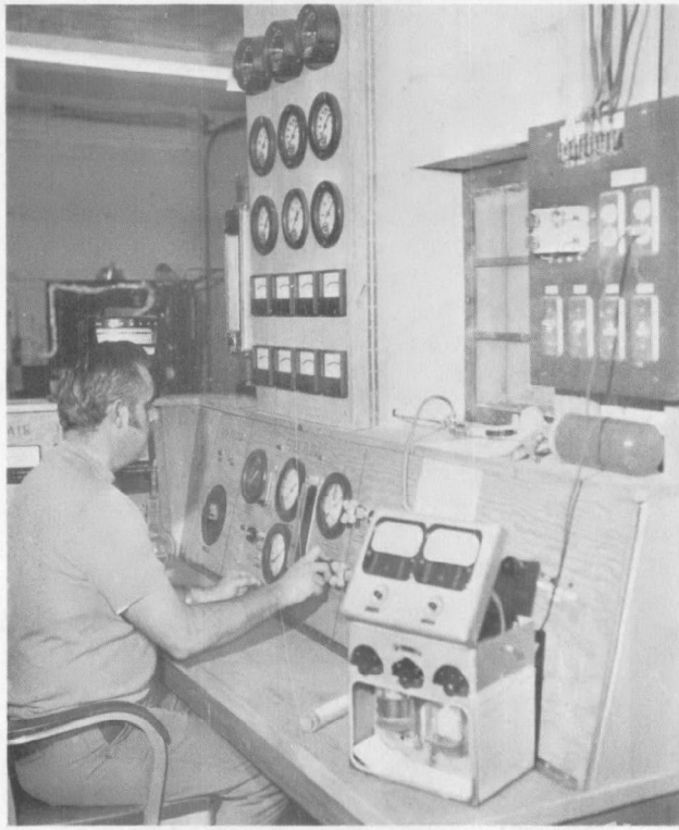
A. Console for Burner and Component Test Facility (Test Stand Two)
